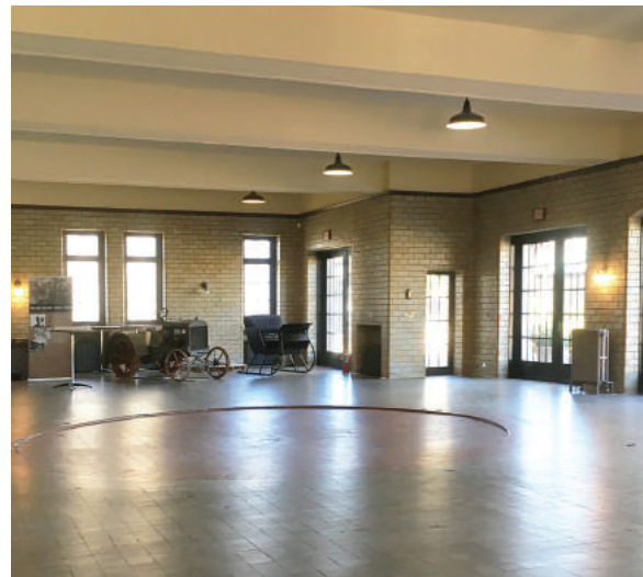
Existing Garage Interior
