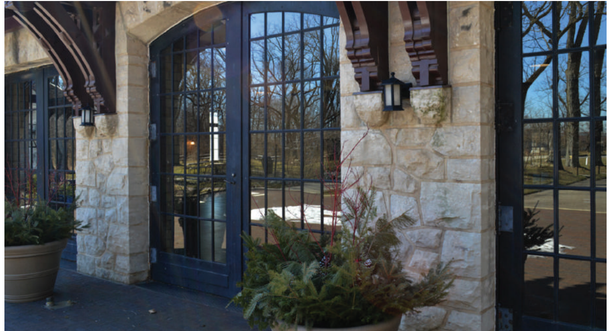
Double Entry Door to Garage
